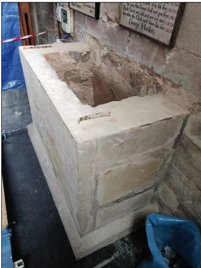
Plate 4: Following removal of the top slab
